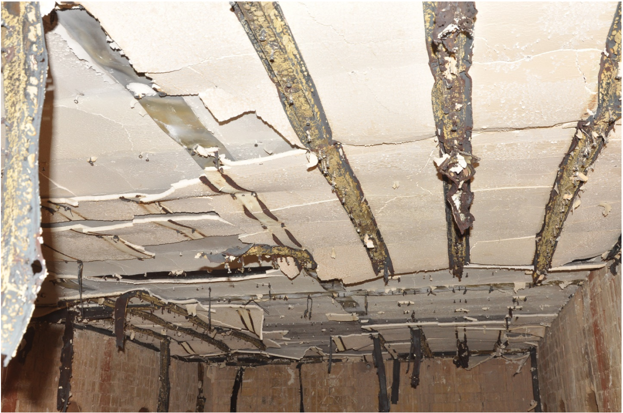
Figure 3.9: Exposed side of specimen after conclusion of the test
