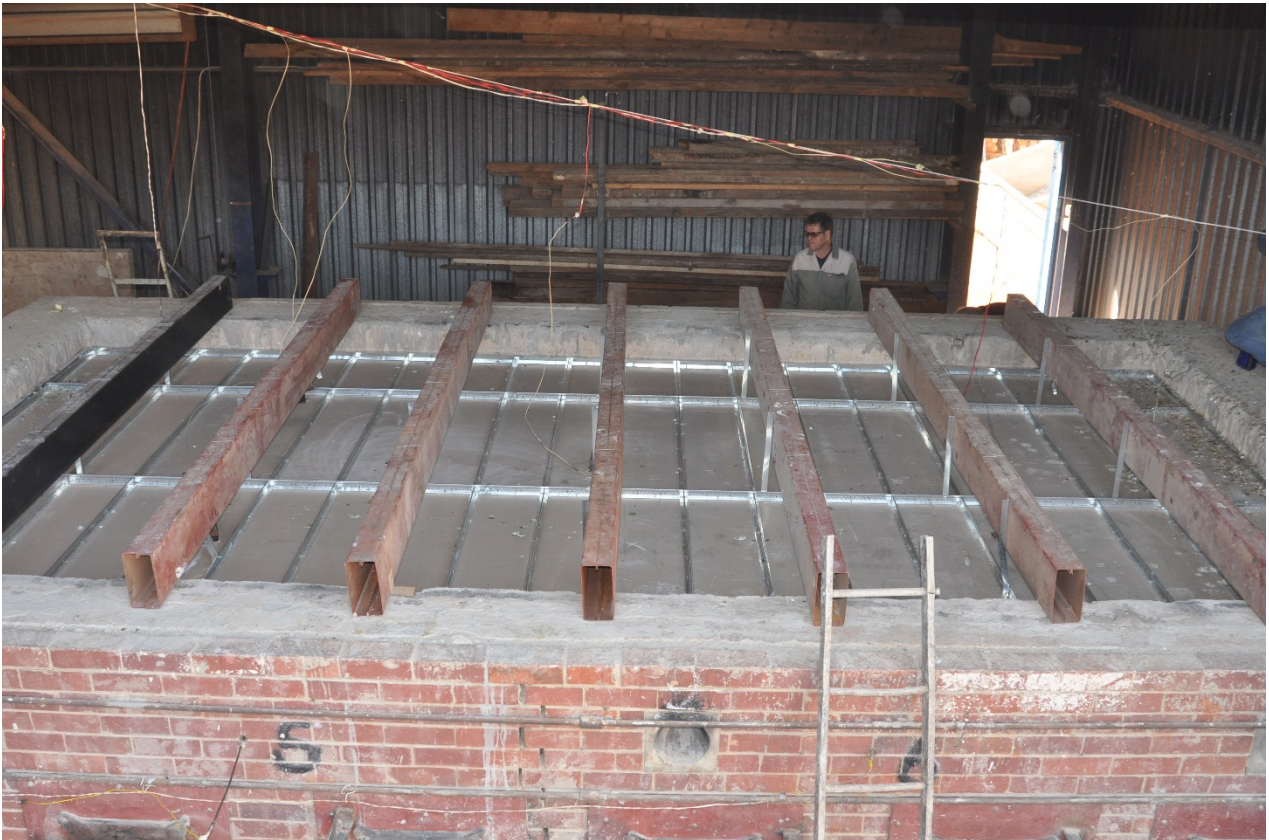
Figure 1.1: The FireShield Ceiling system from the unexposed side prior to the test
