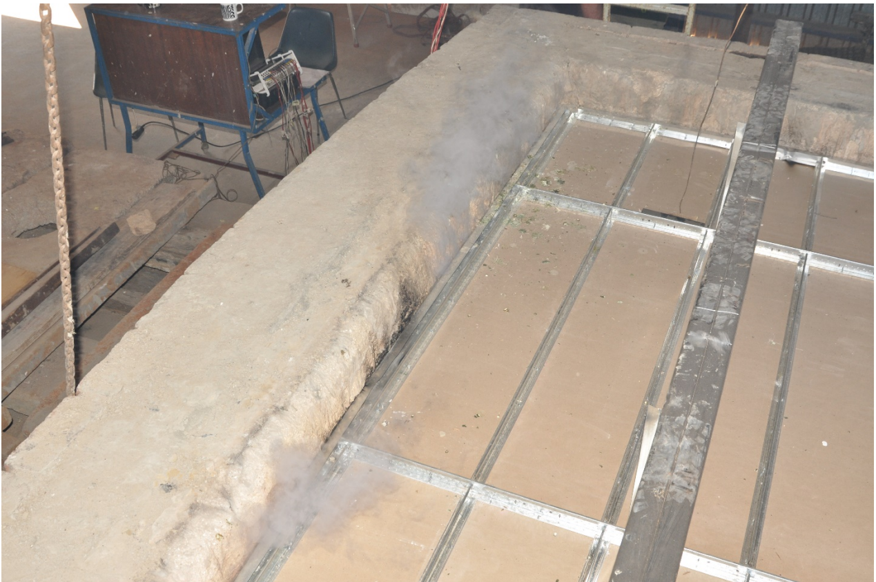
Figure 3.4: Smoke release on the perimeter
