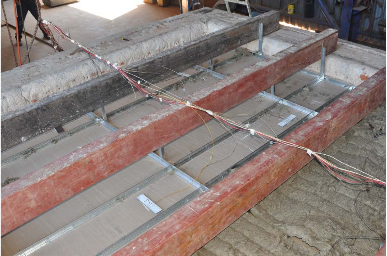
Figure 1.1: The Capco (Uninsulated) Ceiling with thermocouples on the unexposed side prior to testing
