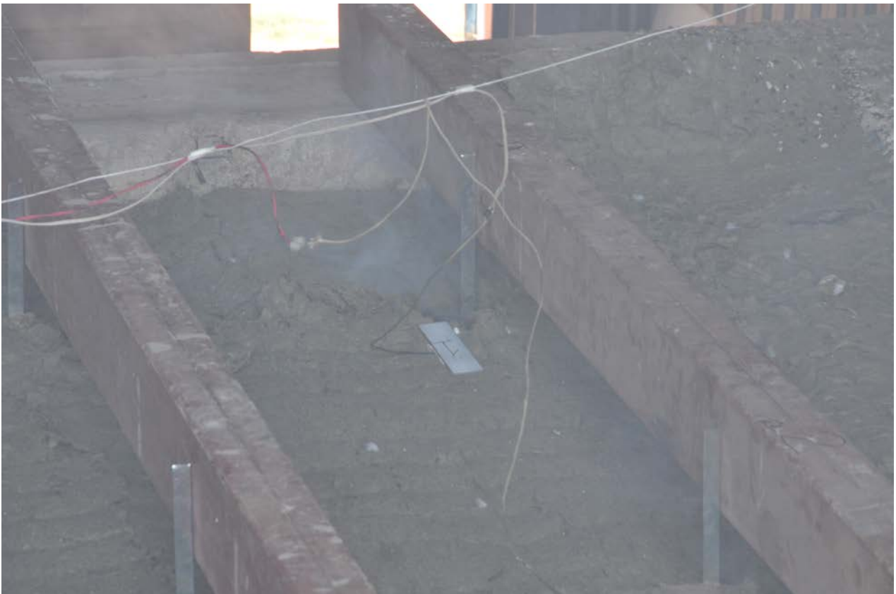
Figure 3.6: Significant smoke release near TC 1
