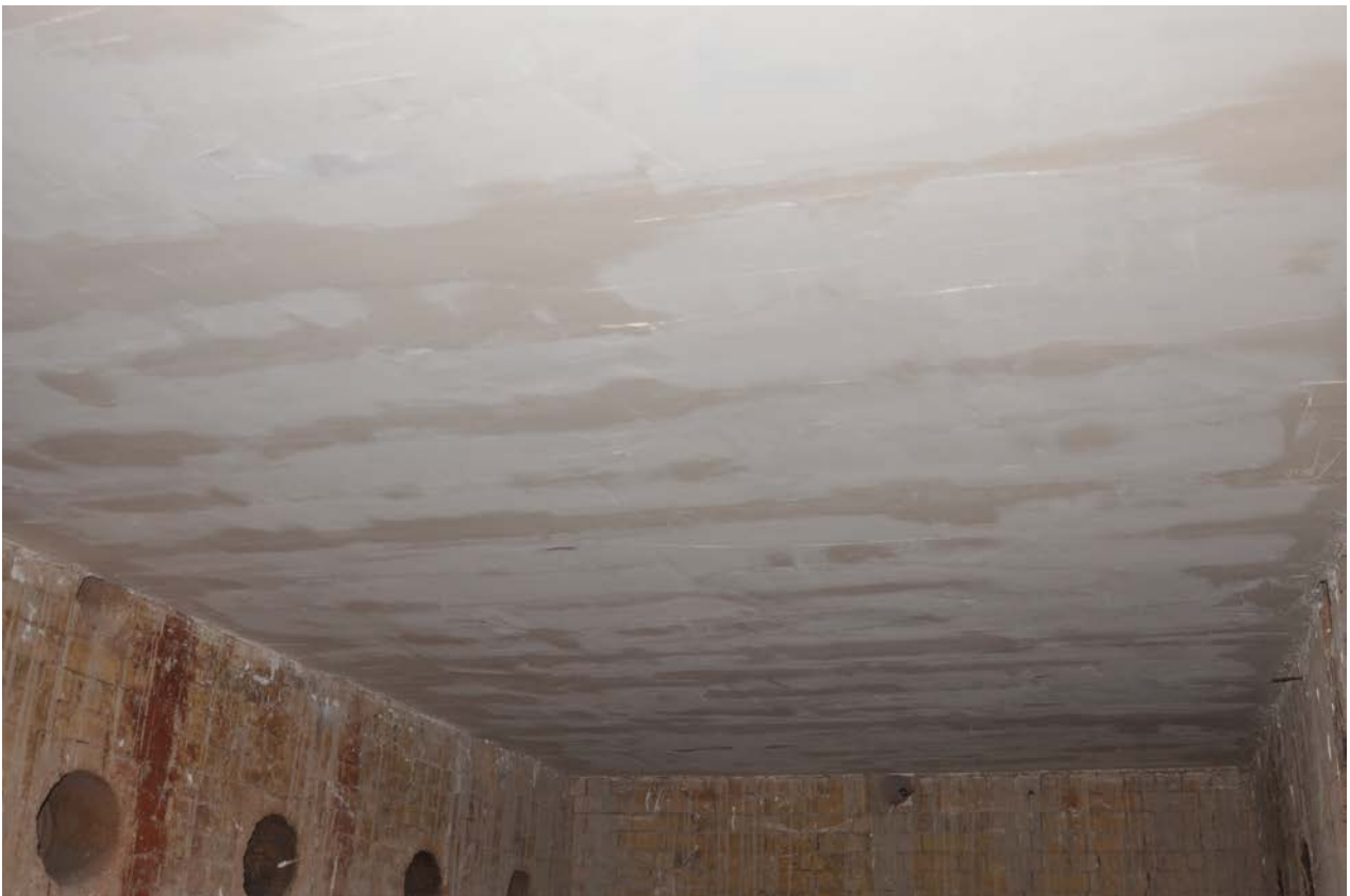
Figure 1.2: The Capco (Insulated) Ceiling from the exposed side
