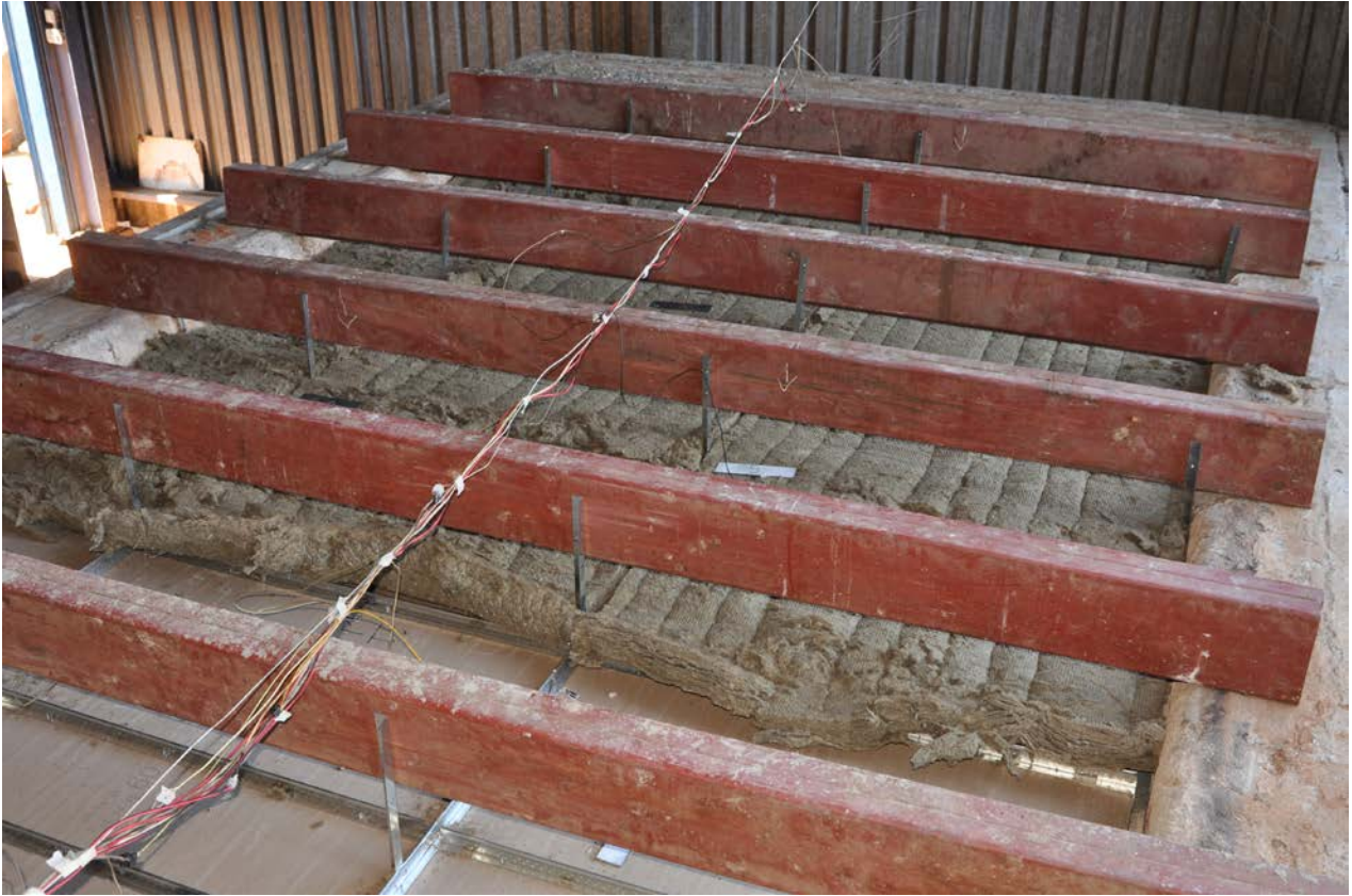
Figure 1.1: The Capco (Insulated) Ceiling with thermocouples on the unexposed side prior to testing
