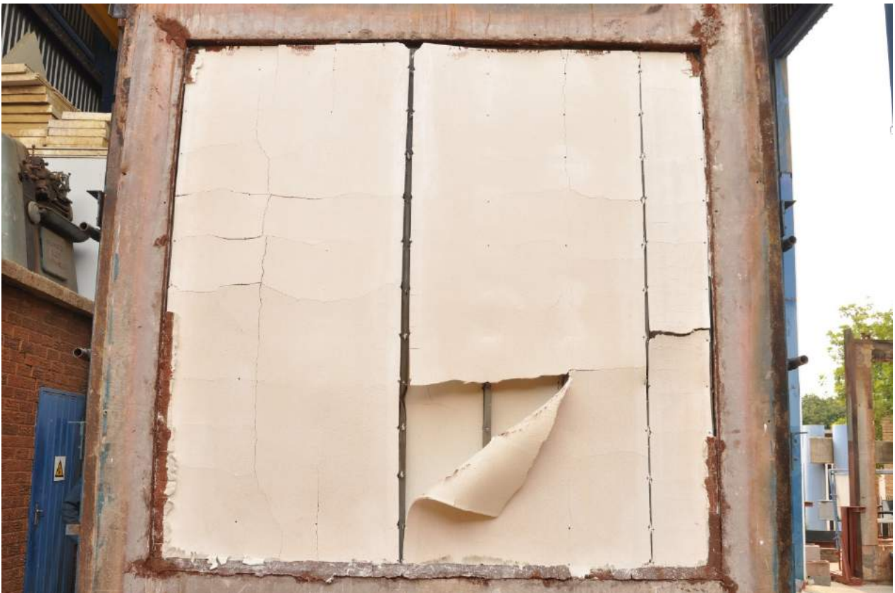
Figure 3.13: Exposed side of specimen wall after removal from SANS 10177 – 2 facility
