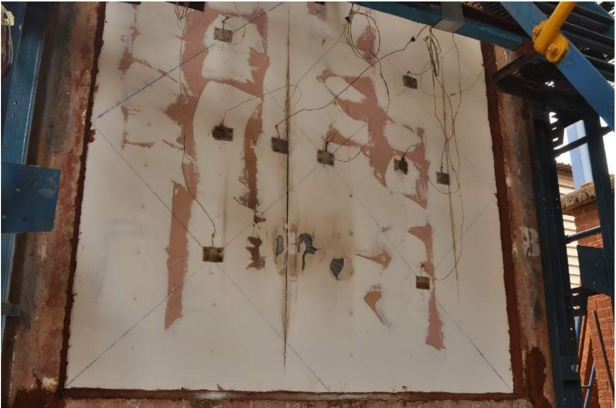
Figure 3.14: Unexposed side of specimen wall after removal from SANS 10177 – 2 facility
