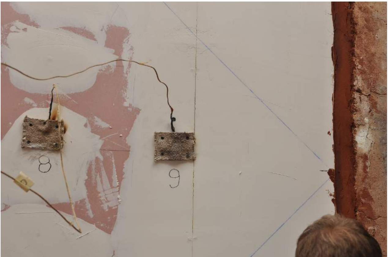
Figure 3.9: Crack forming and discolour on RHJ
