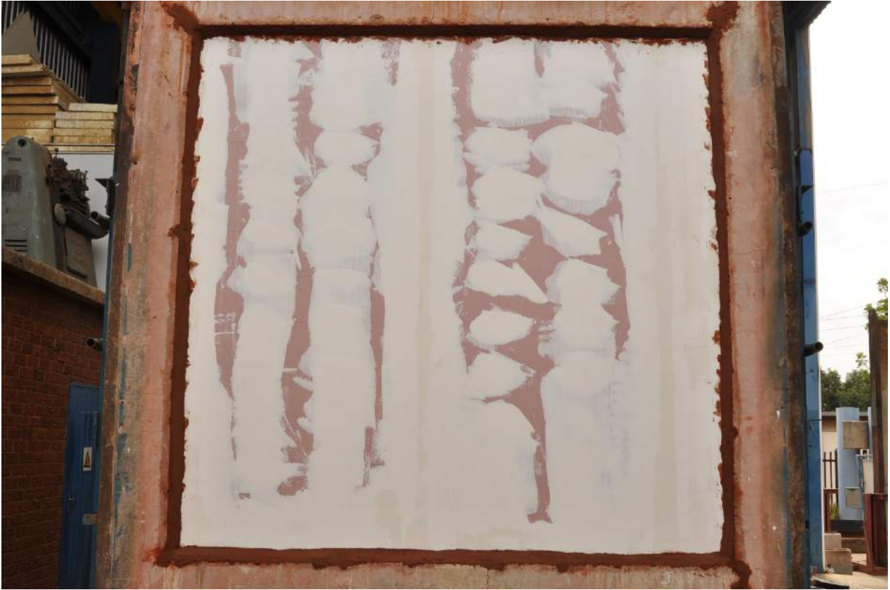
Figure 1.1: FireShield (400 mm stud spacing) system from the exposed side prior to the test
