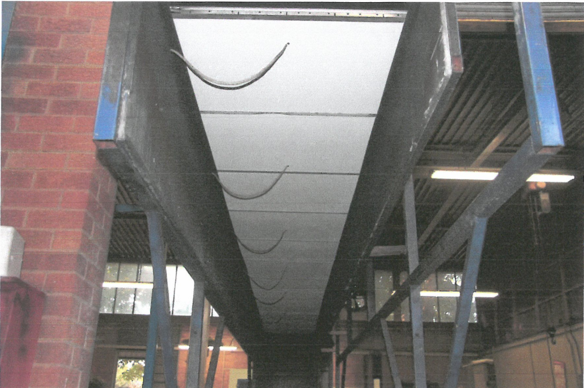
Figure 3.2.1: The test installation prior to ignition of the fire source
