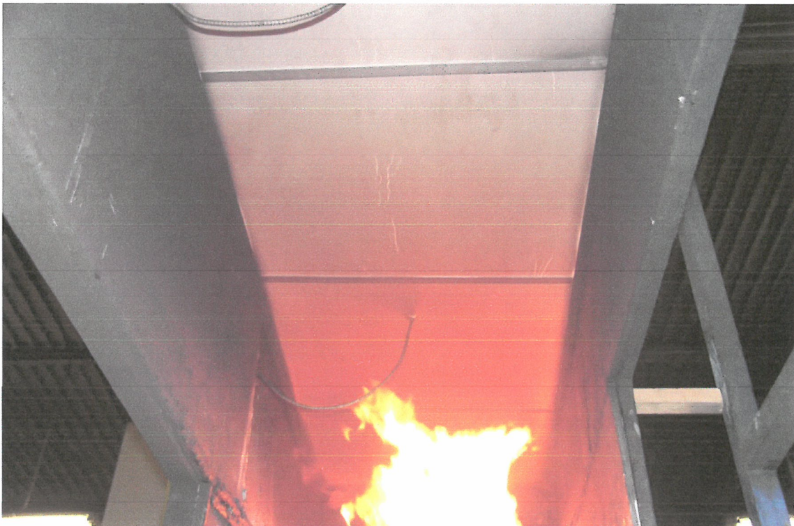
Figure 3.2.2: Cracks visible on the surface coating of the ceiling tiles
