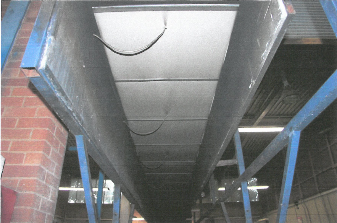
Figure 3.2.3: Test installation subsequent to conclusion of test
